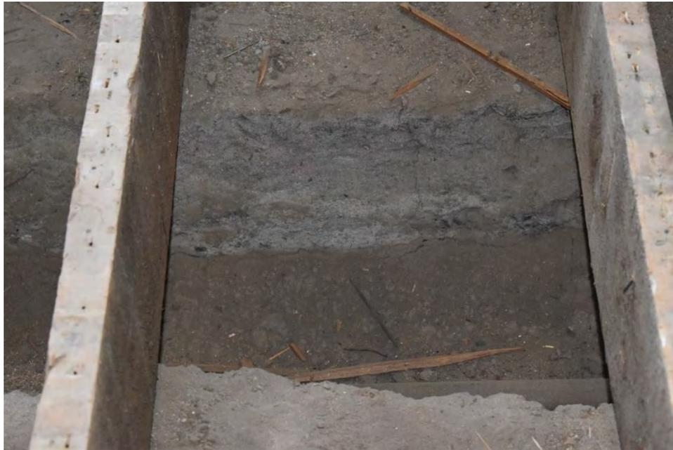
Figure 34. Example of a gas line trench profile.
