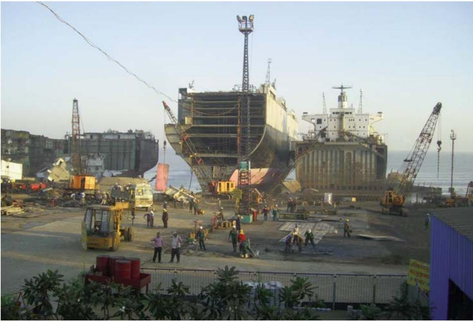
**An upgraded recycling facility. Note concrete aprons, hard hats and modern equipment.**
