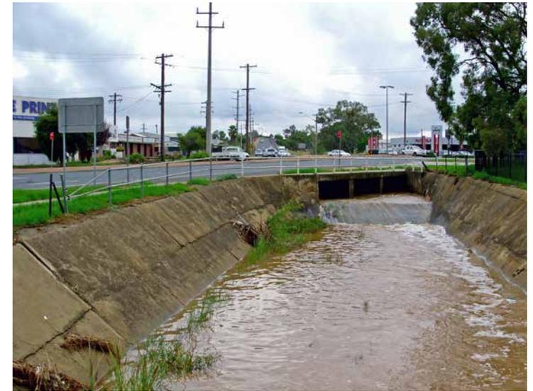
Stormwater in a conventional engineered drainage channel. Source: Bidgee (CC)
